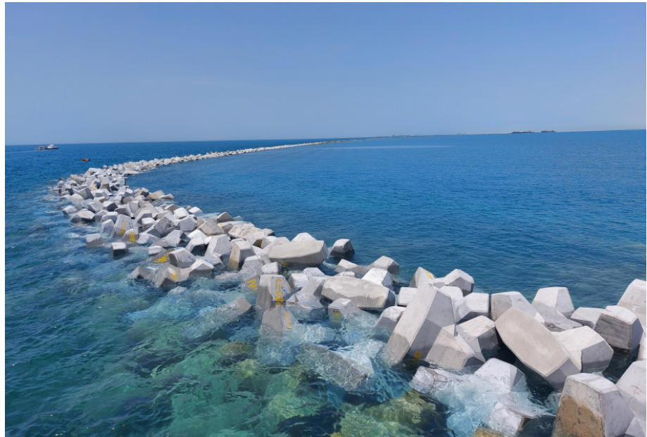
Figure 39: Low-crested breakwater with an ACCROPODE™ I armour facing
