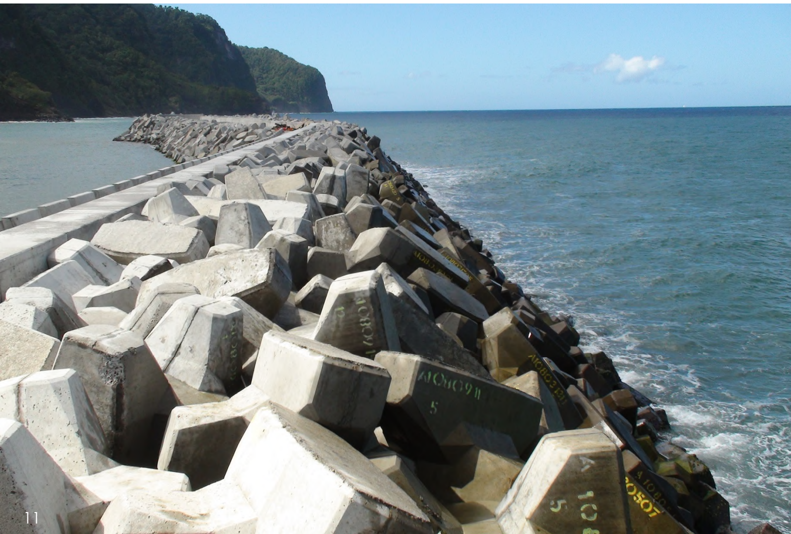
Below - Figure 7: Breakwater with ACCROPODE™ I units - view from the pedestrian walkway on the crest – fishing harbour in Martinique, France
