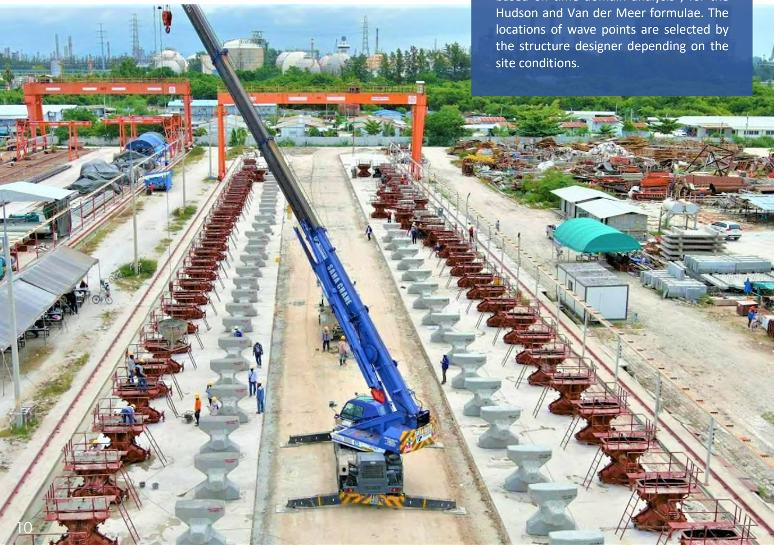
Figure 5: ACCROPODE™ I unit fabrication yard equipped with bridge and mobile cranes
