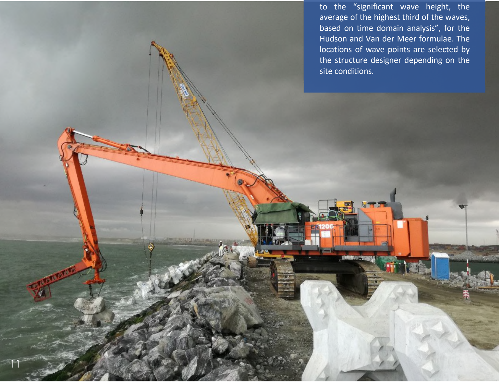
Figure 6: Hydraulic shovel and lattice boom crawler crane during ACCROPODE™ II unit placing
