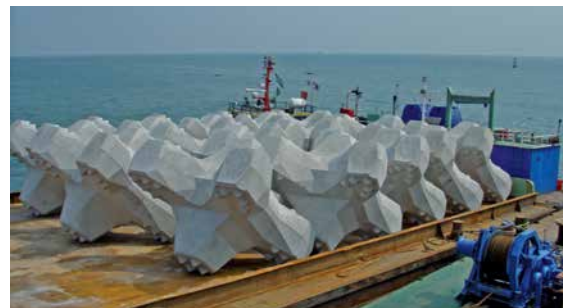
Transport by barge
