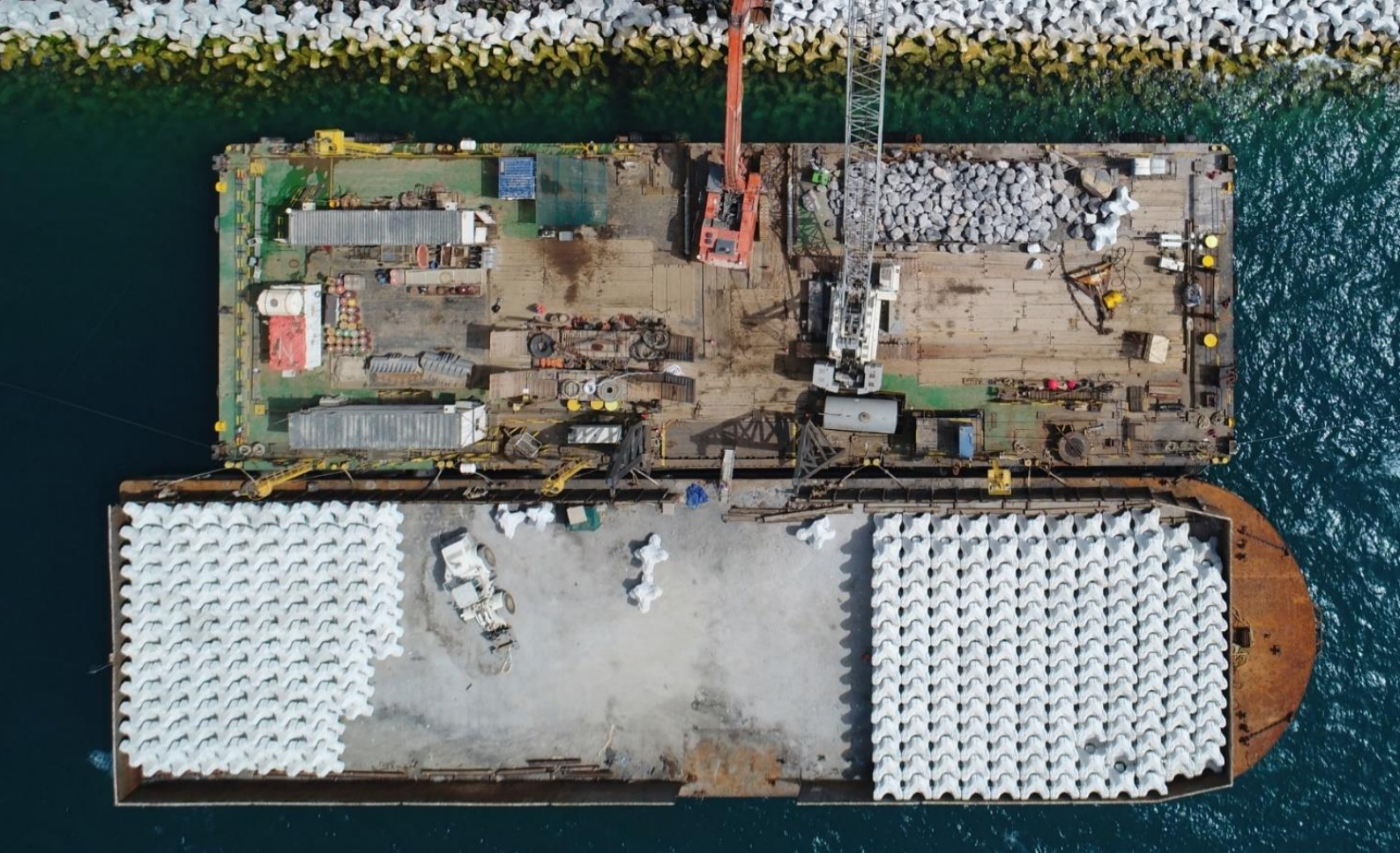
Figure 10: photograph of ACCROPODE™ unit placing using a crane mounted on a barge
