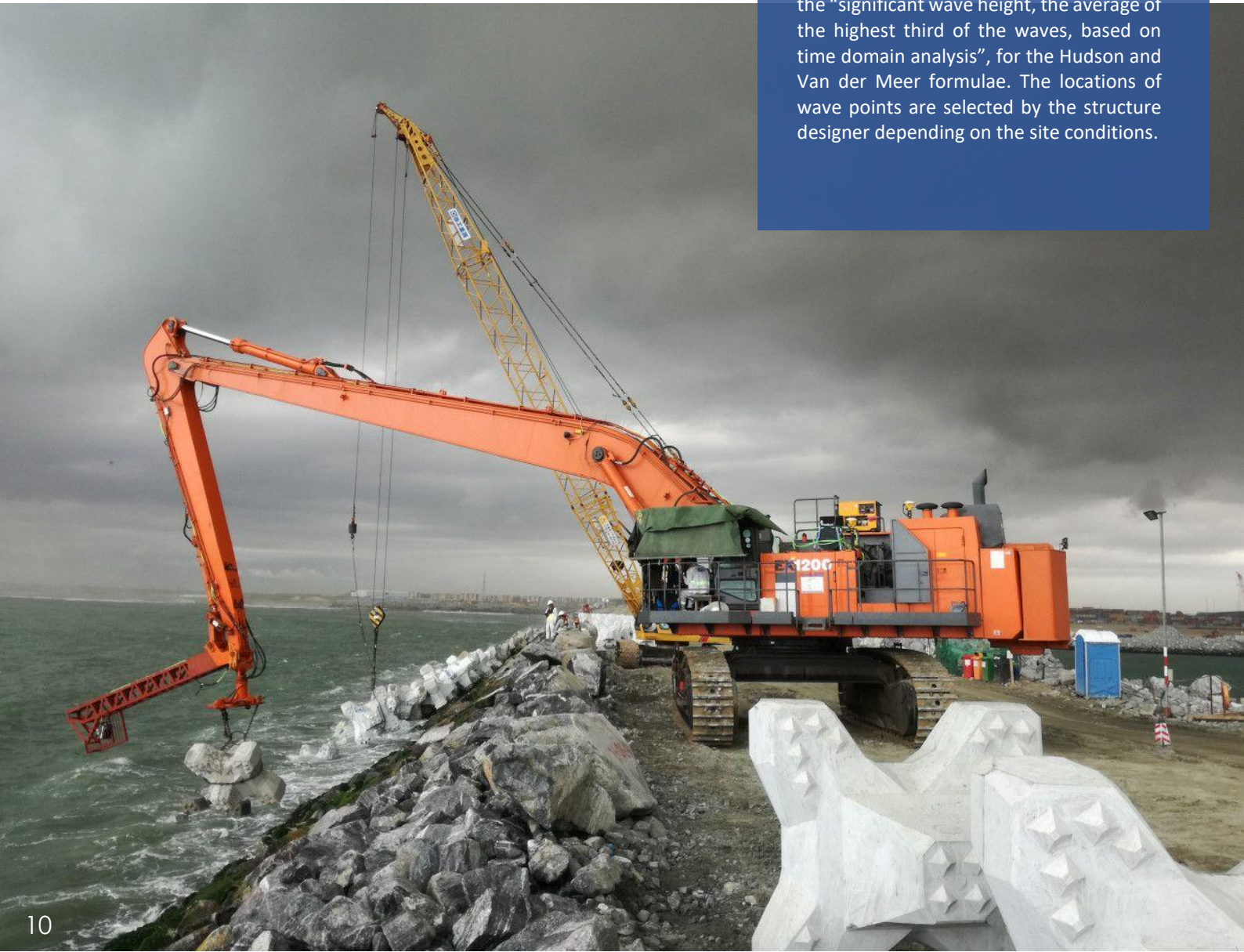
Figure 5: Hydraulic shovel and lattice boom crawler crane during ACCROPODE™ II unit placing
