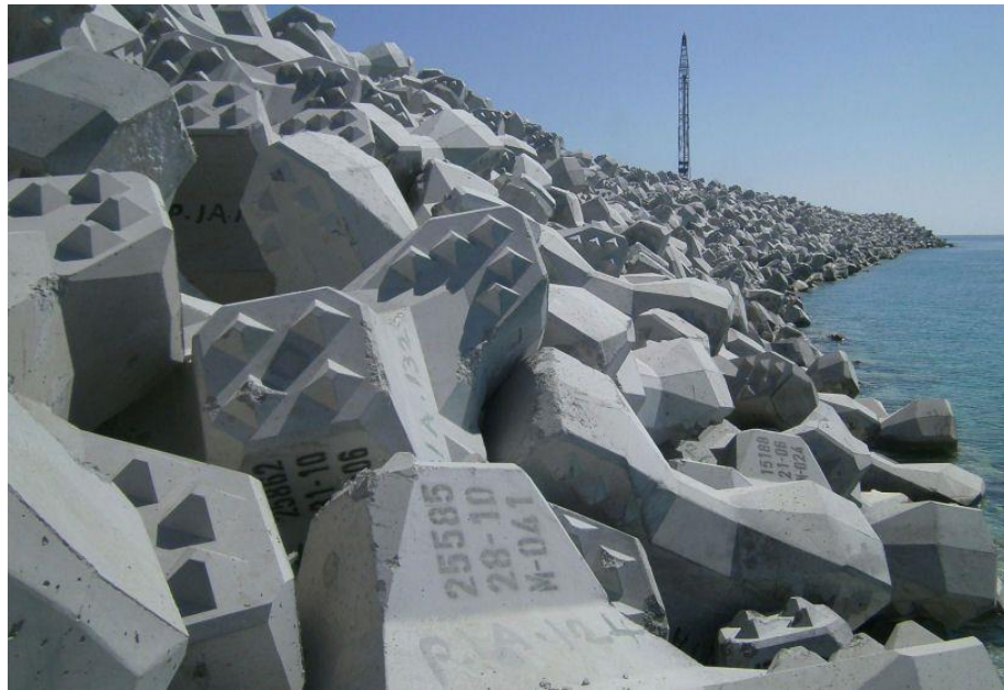
Figure 42: Upper Zakum project in the United Arab Emirates
