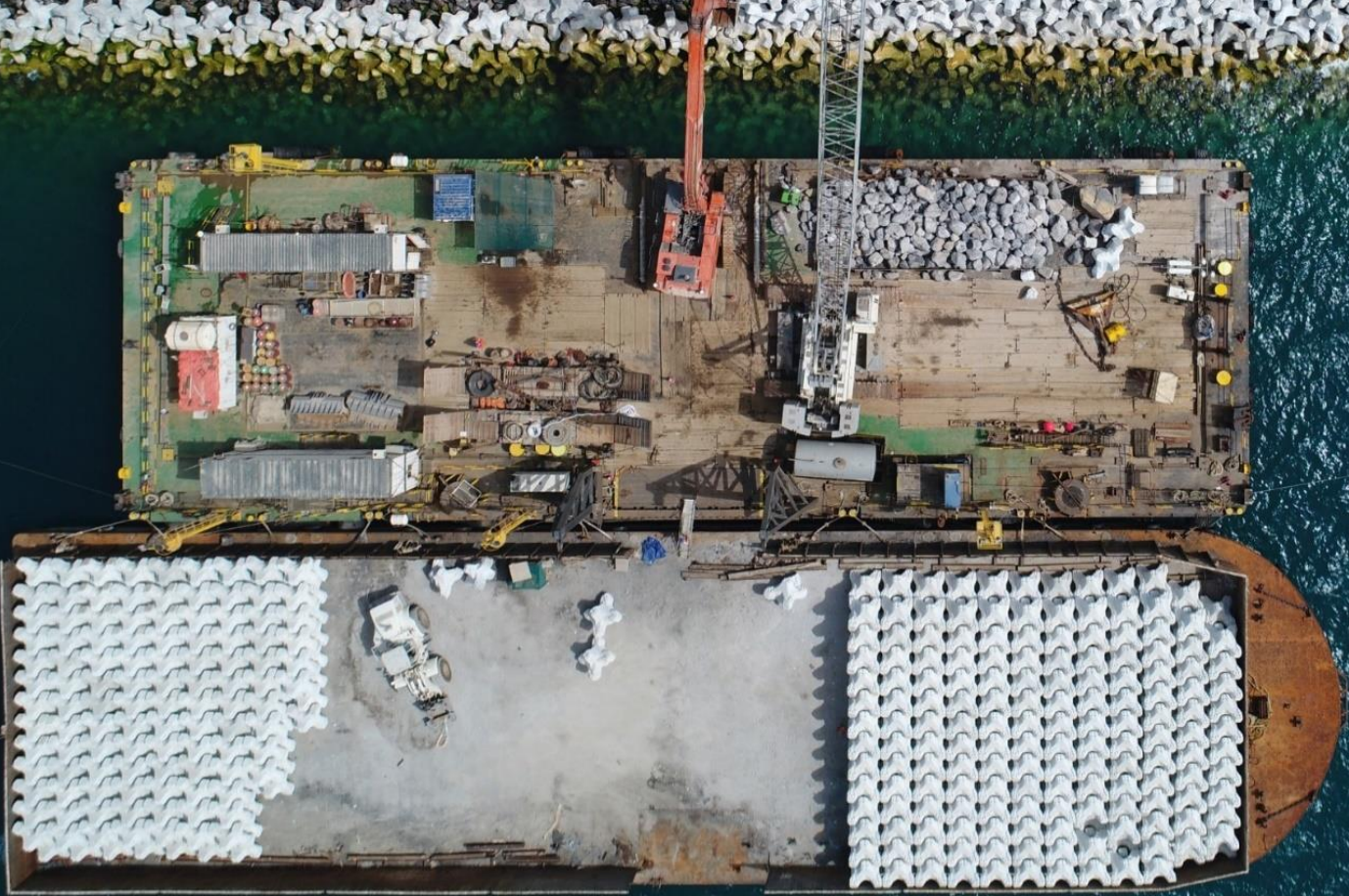
Figure 10: photograph of ACCROPODE™ unit placing using a crane mounted on a barge
