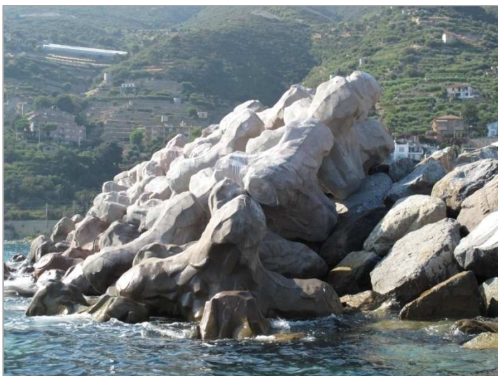
Above water ECOPODE™ armour in progress
