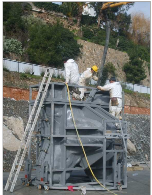
Casting using a chute
