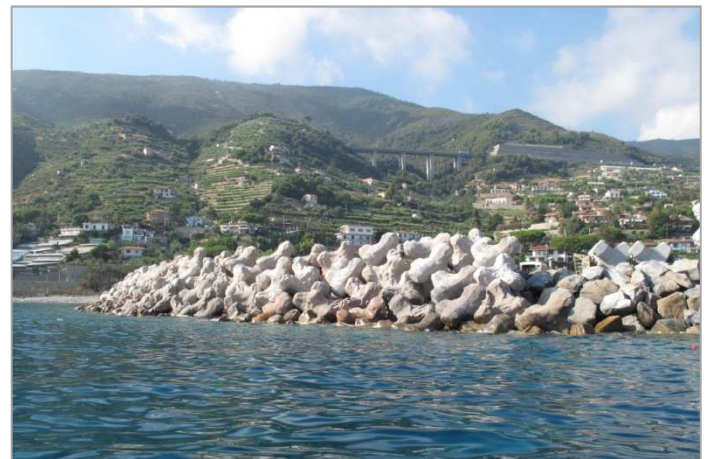
6 m 3 ECOPODE™ units placement in progress
