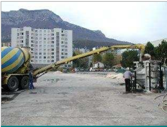
Casting with a conveyor belt
