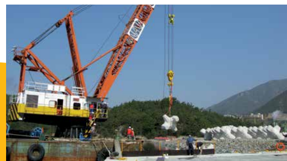
Placement using a floating crane
