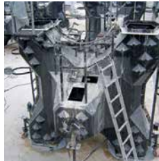
Mould ready for casting
