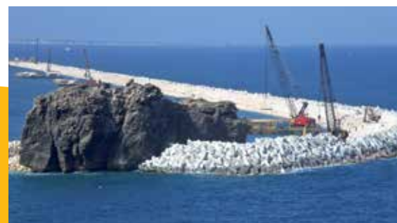
Armouring being completed
