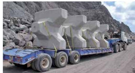
Hauling large units with a low trailer
