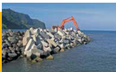
Side view of single layer under construction
