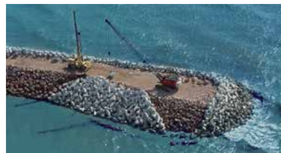
Placement in progress
