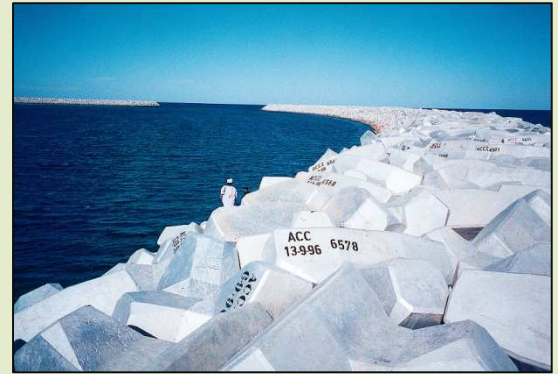
Harbour protected by ACCROPODE™ units
